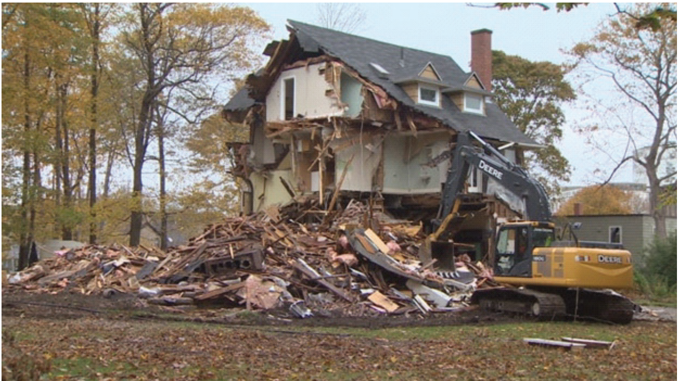
Image 1: Five-unit Arts and Crafts style Campbell home, 825 Young Avenue, designed by Canada's then foremost architect Edmund Burke 1902, demolished in 2016. (CBC)
